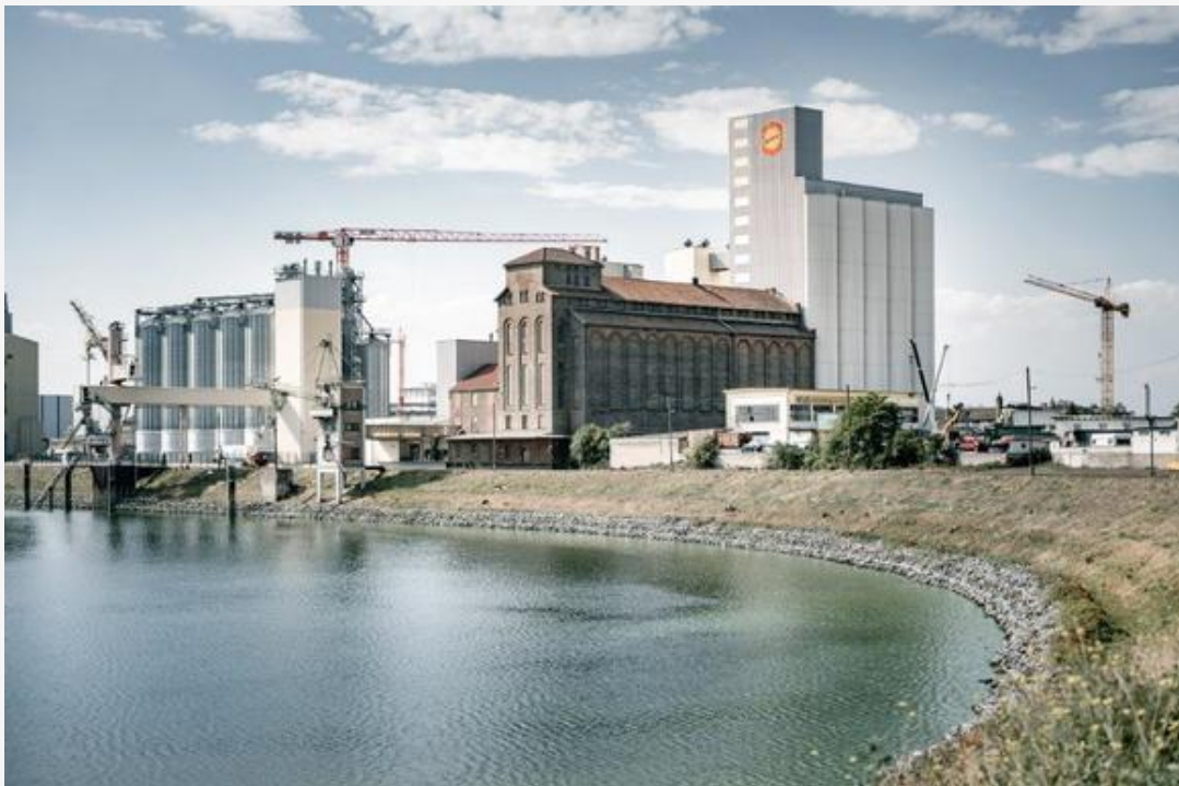
GoodMills Germany production plant - Hildebrandmühle Mannheim -
